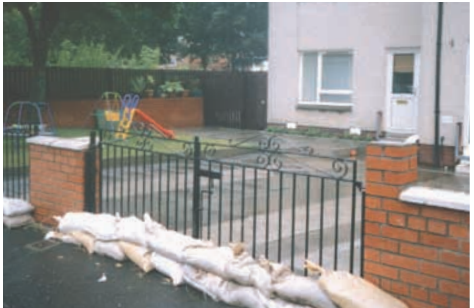
Flood prevention measures in place in Sandyhills.
